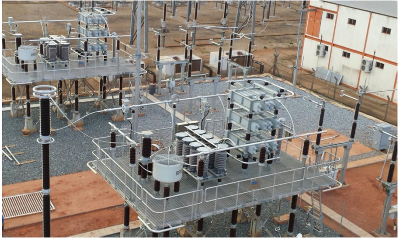
EPC: EdM 3x 220kV Series Compensation
