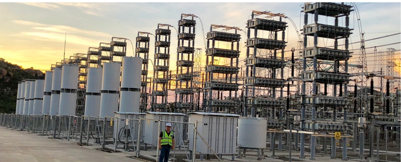
EPC: HCB 220kV AC Harmonic Filter Banks
