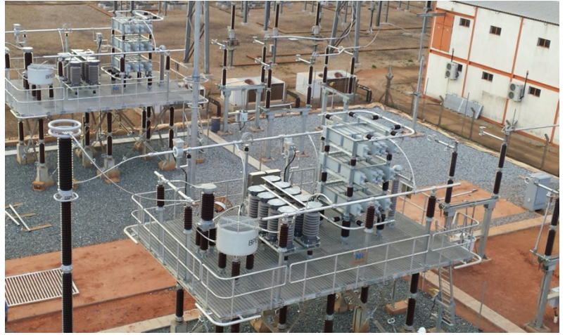
EPC: EdM 3x 220kV Series Compensation
