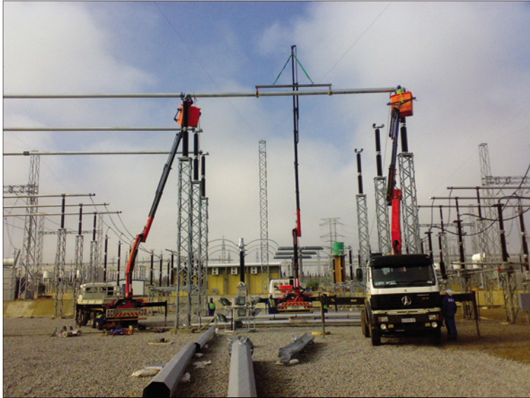
Fig. 5: Installing tubular busbars.
