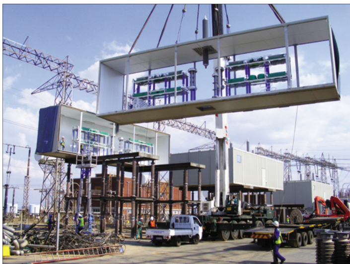
Fig. 3: Lifting a pre-assembled capacitor bank into place.
