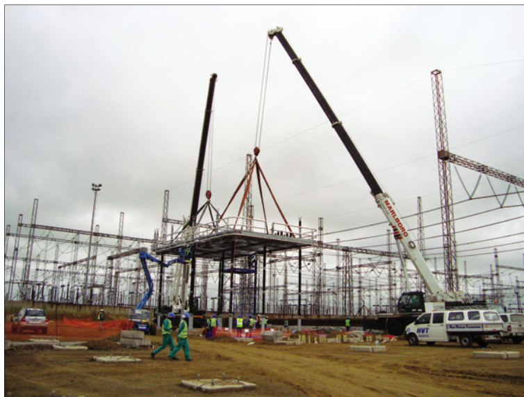
Fig. 2: Correct sized cranes makes work safer and faster.
